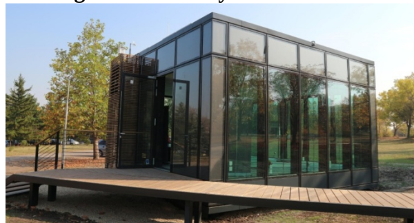
Fig. 2. InDeWaG Demonstation Pavilion, Sofia, Bulgaia
