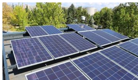
Figure 2. PV system on the roof of the innovative demonstrational pavilion in Sofia with installed capacity 5.04 kWp
